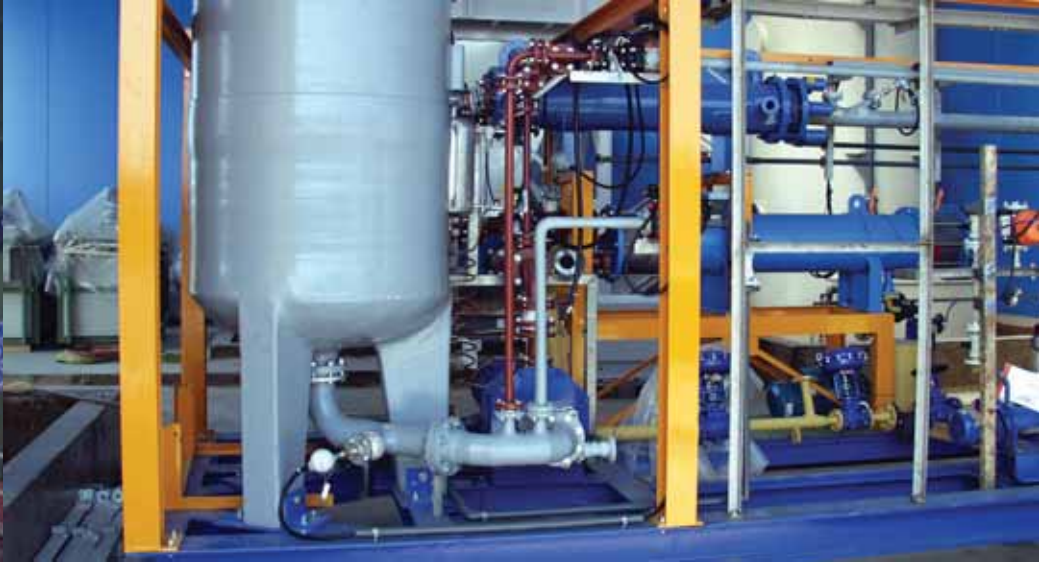
^ Treatment and recycling of expended solutions from the chemical pre-treatment unit.
